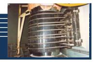
Antiwhip devices and crushable devices for secondary pipes, VVP (steam) and ARE (Feed water) for nuclear island of nuclear power plant.
