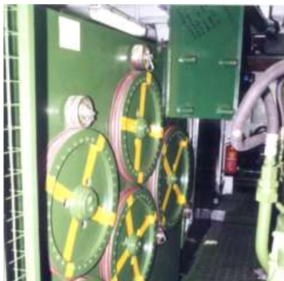
20 T. COBRA winch on board RRS DISCOVERY
